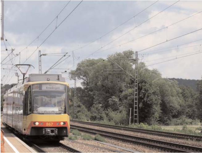
Figure 4 Karlsruhe’s tram-train is a dual-mode vehicle that can be run on tram and train tracks and on AC and DC power, allowing for direct connections between cities and towns and reducing infrastructure costs.
