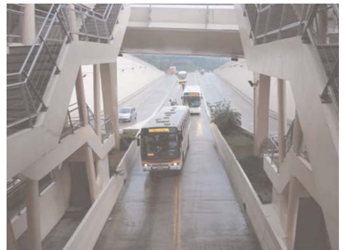
Figure 5 Porto Alegre grade-separated BRT station.
