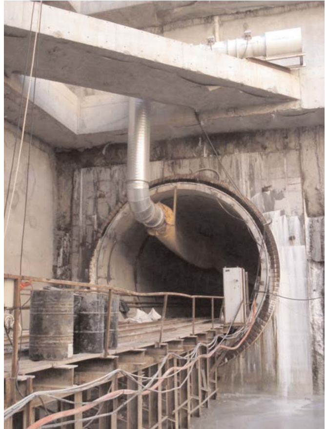
Figure 5 Marmaray tunnel portal.
