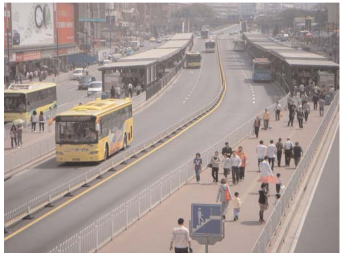
Figure 3 BRT station in Guangzhou.
